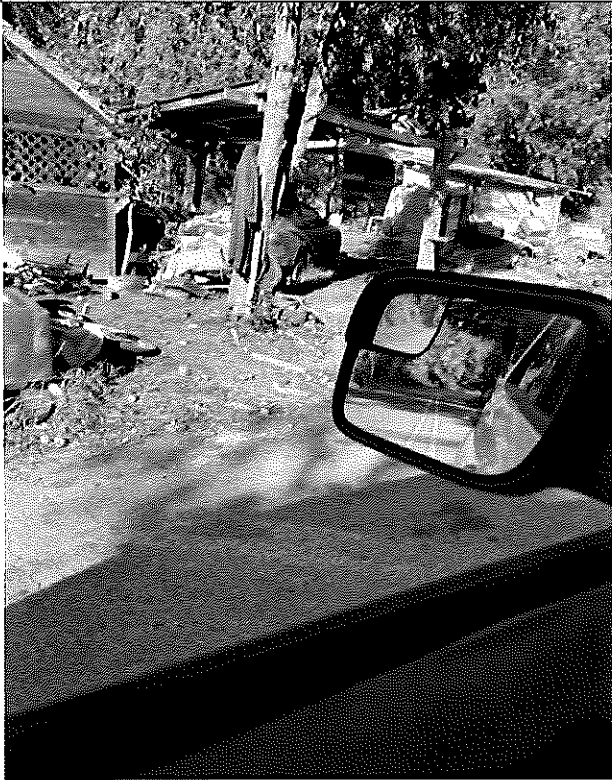
Converted structure to a dwelling without permits
